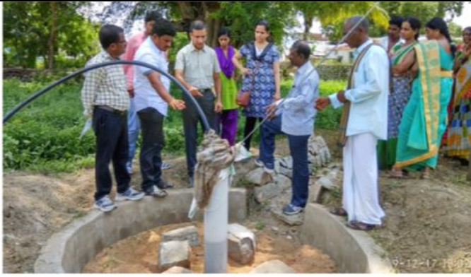
Borewell Recharge structure
